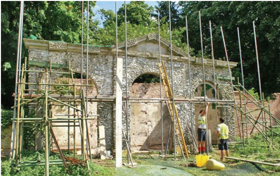
Figure 4 Cobham Aviary, Cobham Park, Kent, undergoing restoration and repair
