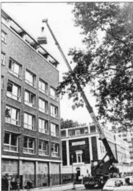
Figure 3 The crate containing the cache of statues suspended from the telescopic crane used to lift it up to the sixth floor of the Institute of Archaeology, London.
