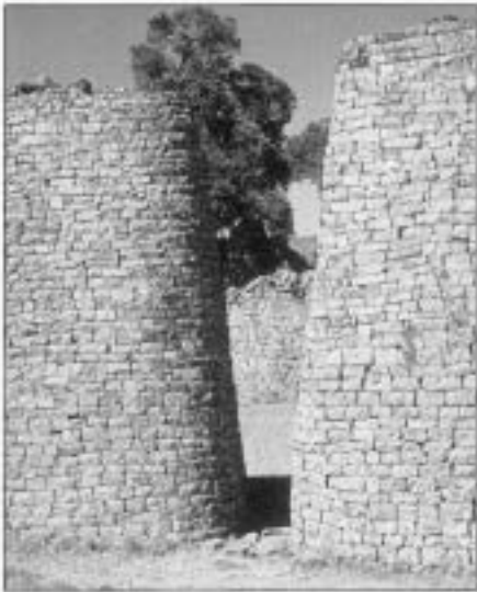
Figure 3 The northeast entrance to the elliptical building at Great Zimbabwe, Zimbabwe.
