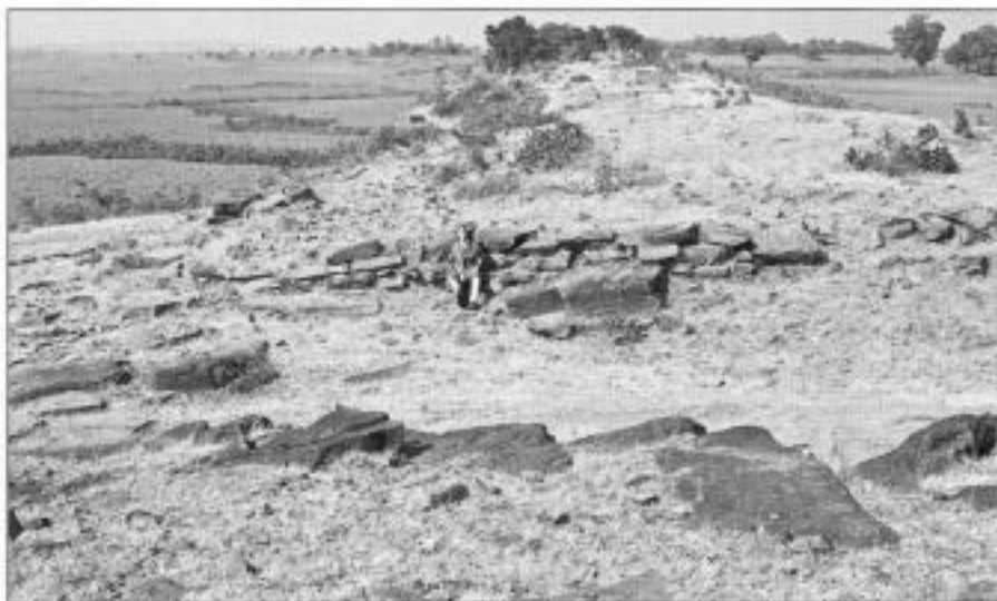
Figure 6 An ancient dam at Devrajpur, with spillway in foreground.
