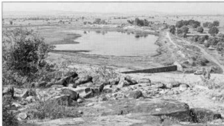
Figure 7 An ancient dam at Chandna, reconstructed in recent years.
