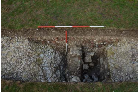
Fig. 7: The wall footings in Trench 11. The main wall cut on the right has been robbed of its stones and the carved chalk blocks of the retaining wall (centre) have collapsed into the resulting void. Note the difference in the disposition of the demolition rubble either side of the wall.
