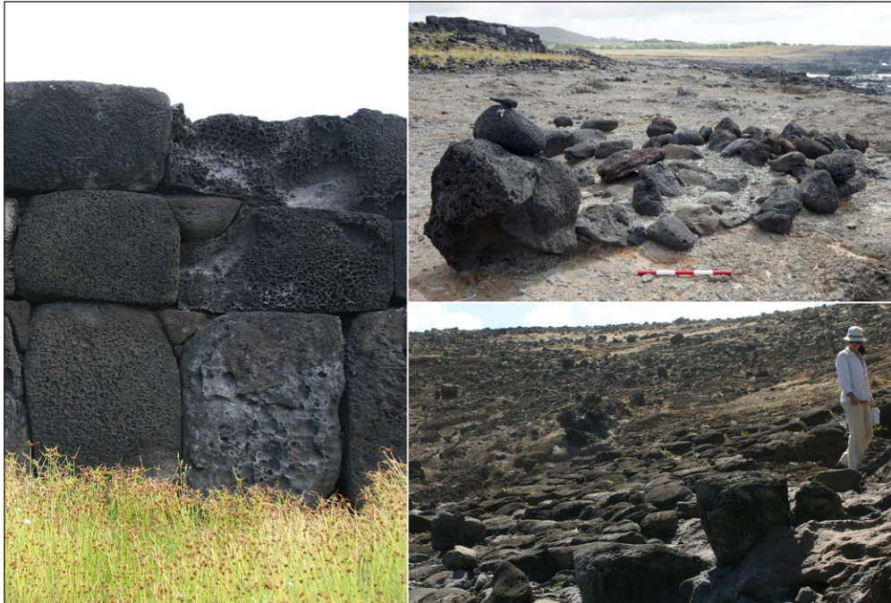
Figure 2: Coastal ahu are open to many threats. Left: tafoni in the rear wall of Ahu Haŋa Poukura caused by the re-crystallization of absorbed salt within the rock. Top right: also to the rear of Ahu Haŋa Poukura, the remains of a sea-washed crematorium. Bottom right: a paved route to a freshwater spring at the shore's edge at Ahu Haŋa Teteŋa, which is being degraded by wave action and by people and animals accessing the spring. Photos: Sue Hamilton (left) & Mike Seager Thomas (right).
