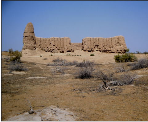
Figure 2: Tumsukly Minara caravansary (Turkmenistan) with central entrance (largely collapsed) and minaret (left). (Photo: Annamyrat Orazov).
