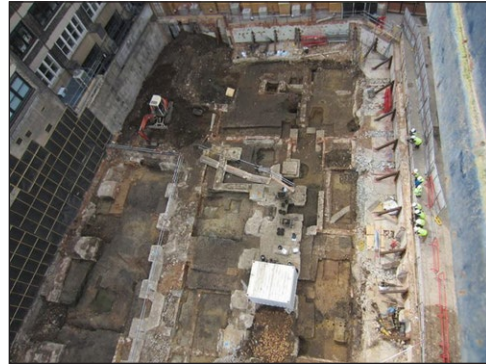
Figure 8: ASE site near the Aldwych, London (Photo: ASE).
