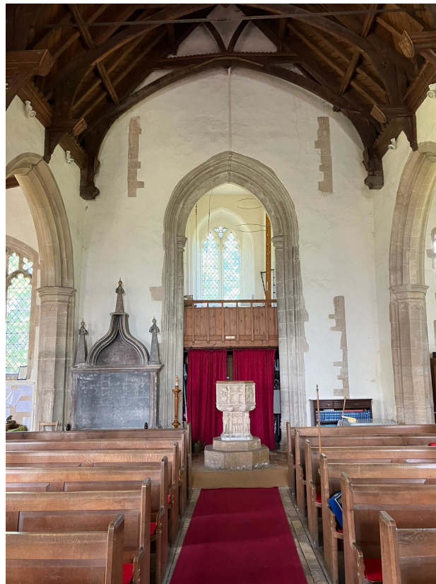
Figure 4 Interior view of St Andrew's Church nave looking west. The diagnostic late Anglo-Saxon long-and-short quoins of the earlier tower are clearly visible in the west wall (Source: Stuart Brookes)
