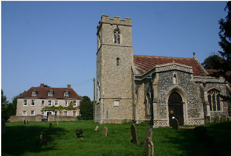
Figure 2 Persistent places in the Suffolk landscape: north-east-facing view of the Old Rectory (left) and St Andrew's Church (right) (Source: © Bob Jones via Geograph.org.uk, CC BY-SA 2.0)
