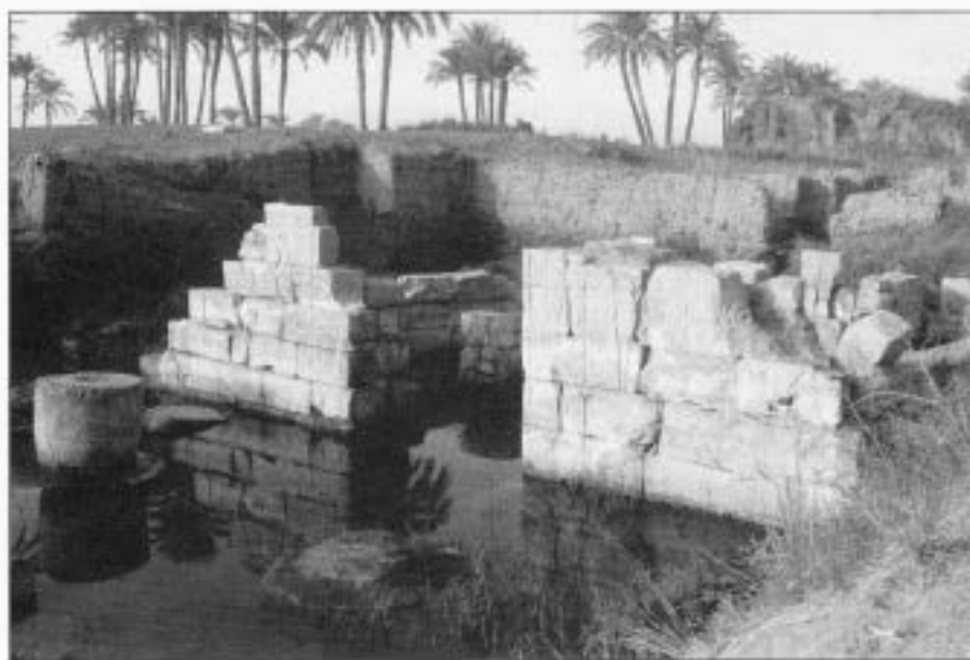
Figure 5 A limestone temple of Ramesses II (thirteenth century BC), one of the monuments at Memphis threatened by rising groundwater and salt damage.
