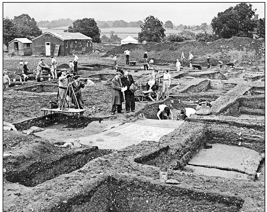
Figure 2 Excavation in progress at Verulamium in 1958, with Maurice Cookson (left) photographing a mosaic floor.
