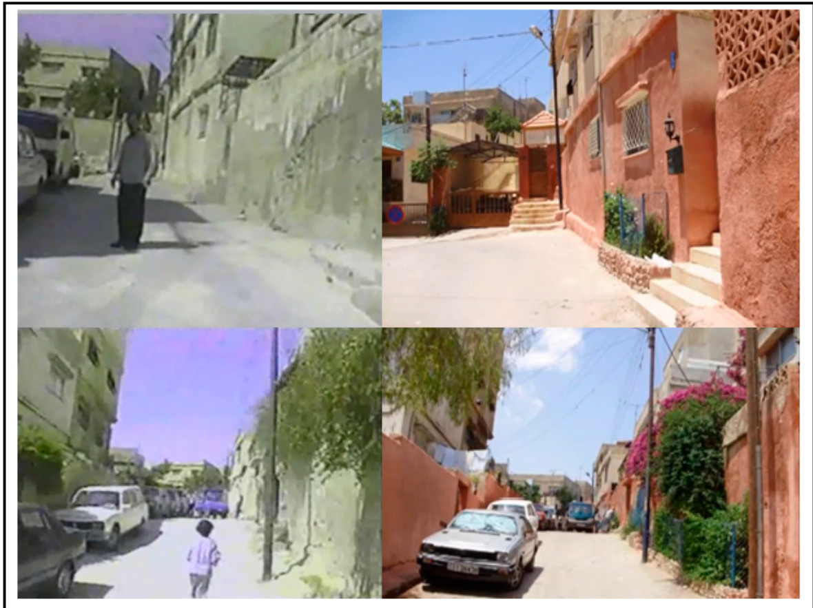
Figure 19 Images of Harra neighbourhoods before (on the left) and after rehabilitation (on the right) (Source: Harra Archive).
