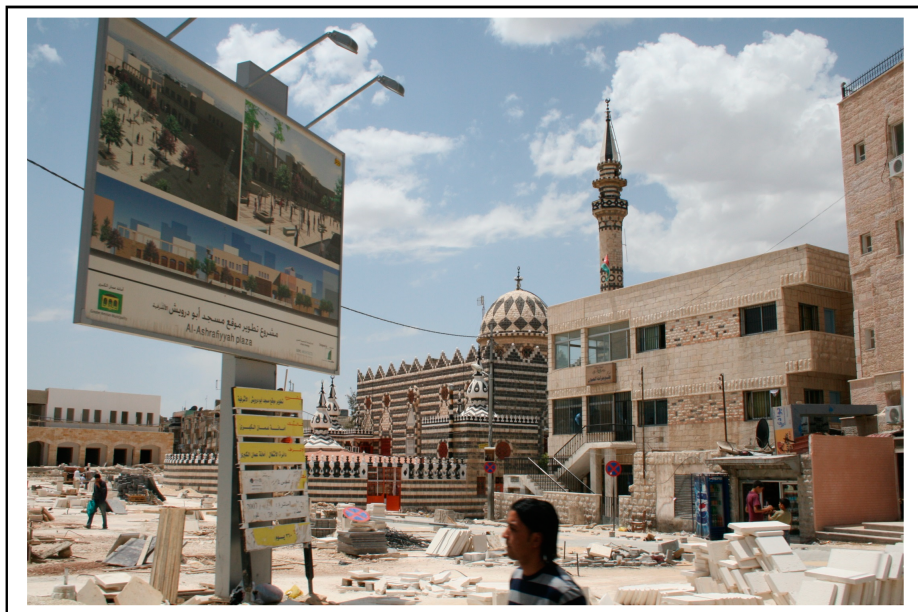
Figure 11 View of Abu Darwish Plaza under construction (Photograph by author, 2009).
