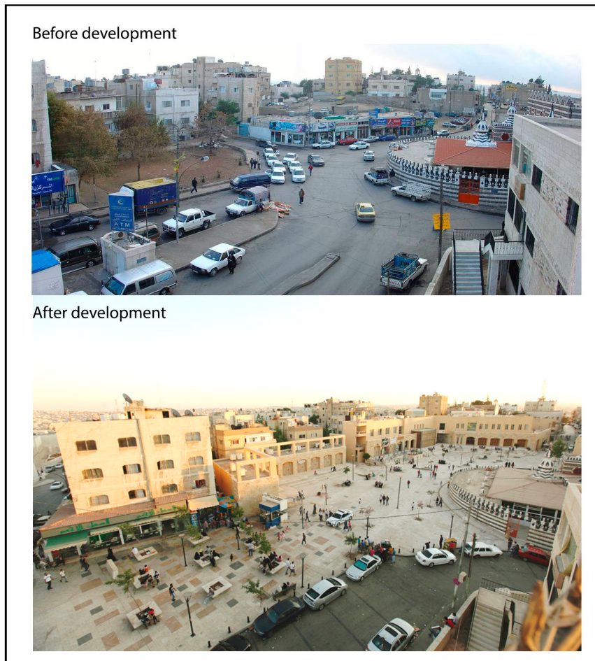
Figure 12 Views of Abu Darwish Plaza before and after development (Source: AB Archive).
