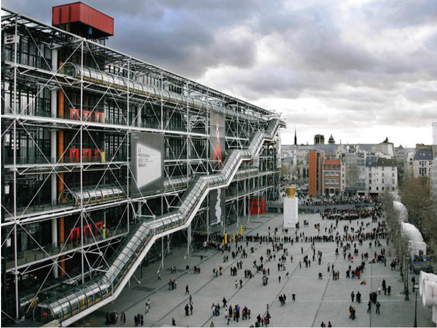
Figure 12. The architects respond to the requirement of polyvalence and plasticity by offering an interior completely empty of its internals. All the service and mechanical systems are transferred in one swooping move to the outside exoskeleton of the building. (estudio campo baeza. Centro Pompidou . Renzo Piano Y Richard Rogers. Photo, October 26, 2012. https://www.flickr.com/photos/campobaeza/8125299099/ )
