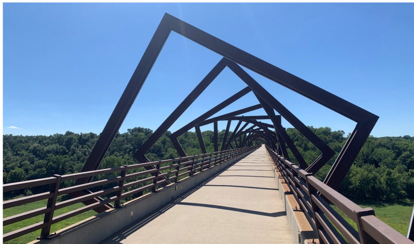
Figure 8. The High Trestle Trail Bridge
