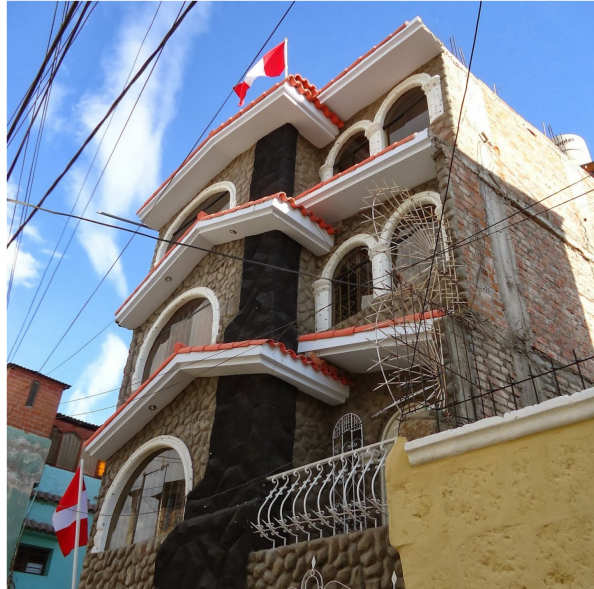
Figure 3. Residential building, Arequipa
