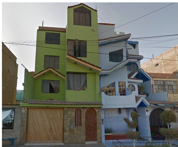
Figure 4. Residential building, Ica
