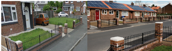
Figure 4: City West Housing Trust “environmental” scheme after works. Source: author.
