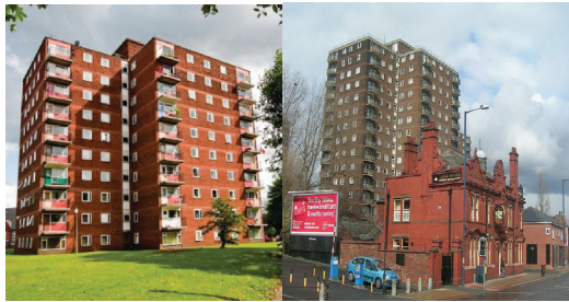
Figure 1: City West Housing Trust high-rise blocks before works. Source: author.
