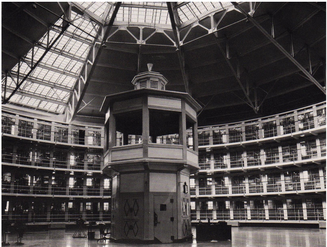
Figure 11: Interior of a cell block at the Stateville Penitentiary near Joliet, Illinois, U S A, W. Carby's Zimmerman architects, 1916-24 (Illinois Department of Corrections)
