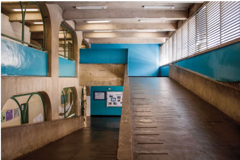
Figure 2 Internal ramps (bottom) linking the three floors of CIEP Doutor Antoine Magarinos Torres Filho, in Rio's Borel district. Image © Aberrant Architecture.
