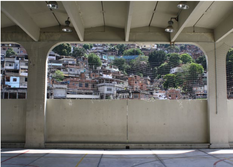
Figure 8 The multipurpose room on the rooftop at CIEP Douror Antoine Magarinos Torres Filho, a compact-designed CIEP. Image © Aberrant Architecture.
