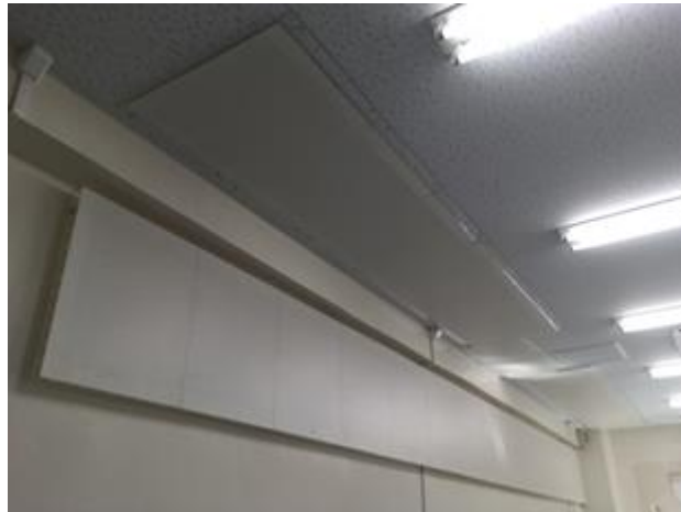
Figure 3. A photograph of a honeycomb-backed box-like MPP absorber panel installed on the corner of the wall and ceiling of a meeting room. The absorber panel is made of plastic sheets and is very light weight. The surface of the MPP is colored with paint, so that it matches with the existing wall. These absorbers are suspended from a picture rail on the wall.
