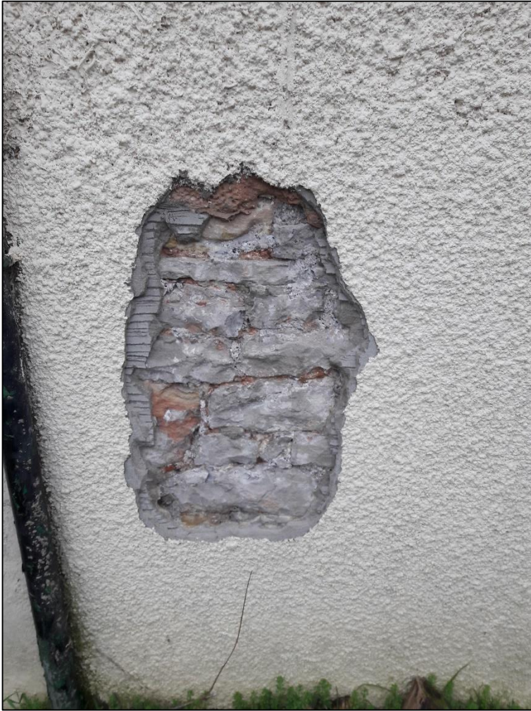
Figure 2: The external face of the pantry wall at Court House showing a rubble wall formed of Sandstone and Limestone blocks with a cement-based, three-coat render system.
